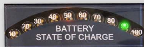
Batteries have a 90% charge
