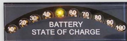
Batteries have a 50% charge
