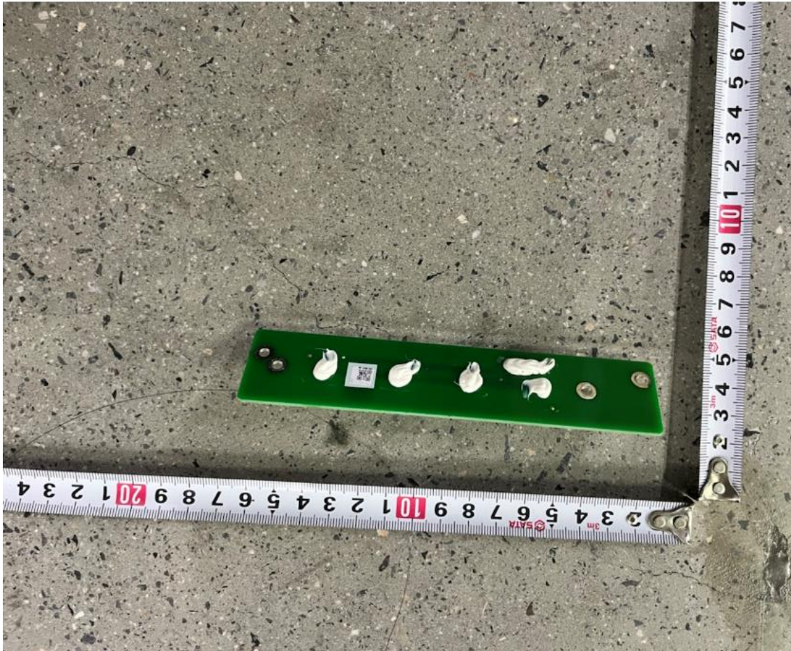
Photo 17: Back view of Lighting board:
